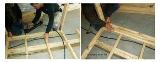
10. Next get a 46 ½ 2x4 and install it between the 1<sup>st</sup> panel and 2<sup>nd</sup> panel, making sure it's up against the floor joist. Nail it in. Then get another 46 ½ 2x4 and place it on top of the one you just installed, laying it flat and line it up with the vertical 2x4's from panel 1 & 2. Nail it in.
