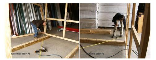
6. Next you will begin to put the other two panels in. First you run a string from the front gable at the bottom to the back gable at the bottom. From the back gable, count two spaces towards the front gable and install the panel in that space. Pull the edge of the panel to within a 32<sup>nd</sup> of the string you installed so that all panels line up even. Then nail it in. You should put at least two nails on each side of the panel when attaching it to the runners.
