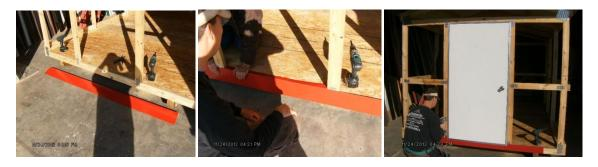
39. Now you will put the dripedge on the bottom edge of the building. Hold the drip edge in place and made proper marks to cut out in metal so that it fits flush onto the bottom edge of the building.
