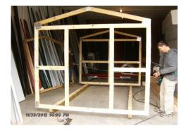
5. Now you must square the building up by measuring from the front right corner gable to the left back corner gable and get your measurement. Then measure from left front of corner gable to right back of corner gable and get the measurement. These two numbers should be the same. If not adjust by sliding one end forward or backward to square up building.
