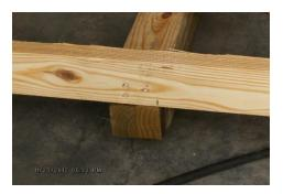
4. Install front gable by doing the same as step 3. Measure over 14" from the end of the gable on both sides. Then slide the gable on the front space of the runner and nail it onto the runners. (Make sure your 14" mark is lined up with the outside of the runner board.)
