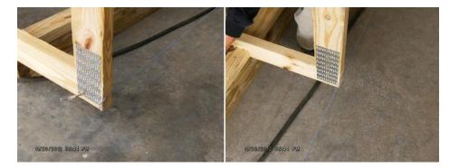
7. Now you are going to put the floor joist in between the panels. Use the spaces between the 14.5" 2x4's. When you lay the joist in the space align the joist so that it's 4 1/4 off the string that you used in the previous step. Once in place, nail it in. You will have 4 joists to install in this step. (Make sure you measure both sides, it should come out to 4 ¼ but you may need to make adjustments if you are off any)
