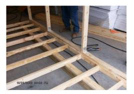
13. Next you will add the 12' 2x6 stripping board down the side of the building. Align it at the bottom of the front gable to the bottom of the back gable. This should be flush at each end. Nail it in. Install nails through 2x6 at front gable, each panel and back gable.
