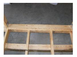
11. Next install the 45 ¾ 2x4 between the 2<sup>nd</sup> panel and back gable, making sure it fits up against the ends of the floor joist. Nail it in. Then get another 45 ¾ 2x4 and place it flat on top on the 2x4 you just installed, lining it up with the vertical 2x4's from the front 2<sup>nd</sup> gable and back gable. Nail it in.
